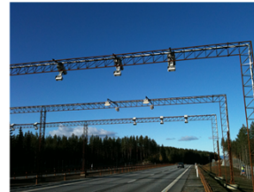
Roadside ITS sub-system
